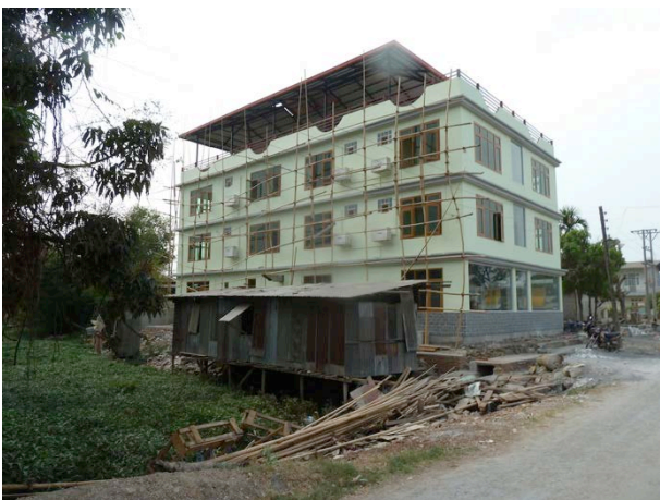
Figure 13: A Hotel under construction in Nyaungshwe
